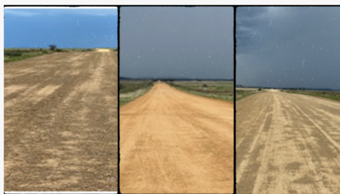
Dawson Road Completed
